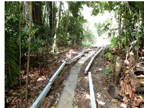
Construction of boardwalk in Windsor Nature Park
